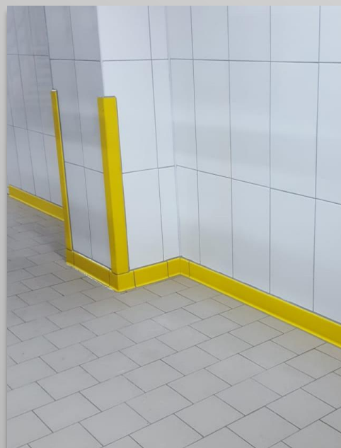
Application de PG-F CORNER
